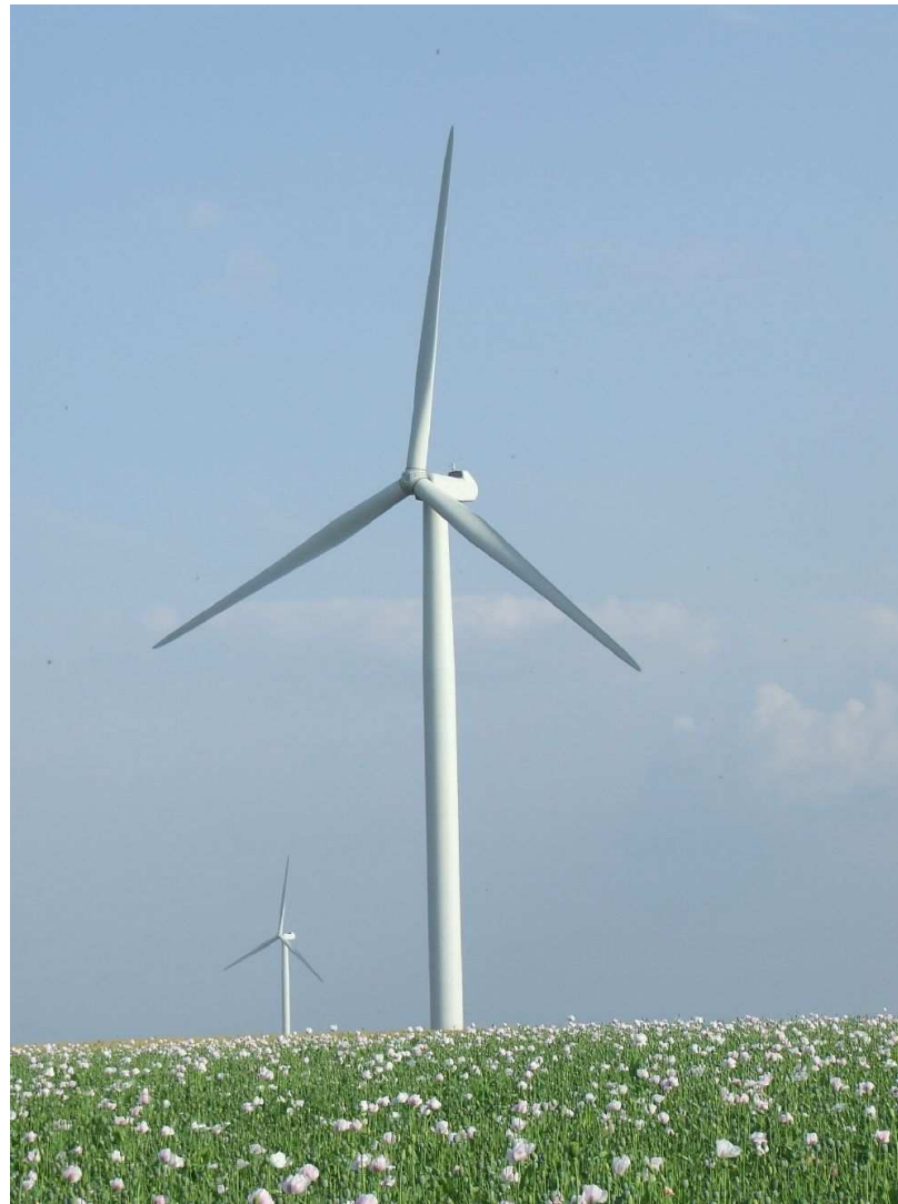
Wind turbine: photo
